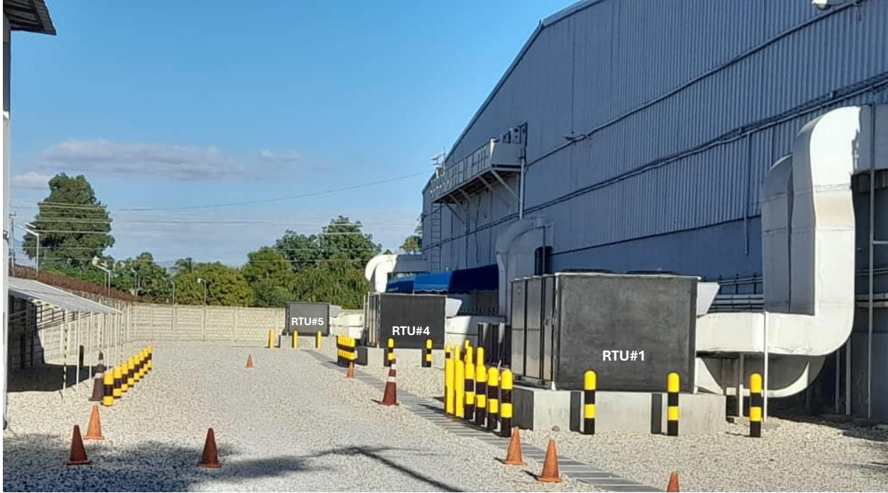
GENERAL VIEW OF THE WAREHOUSE P1
