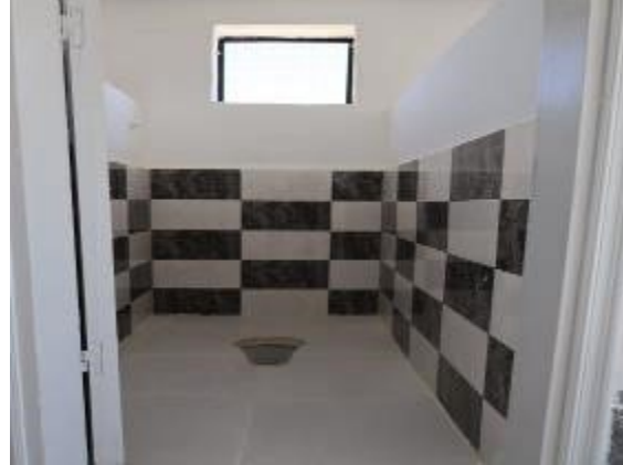
Altali'a Alwusta school post rehab
