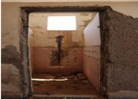
Altali'a Alwusta school prior to rehab
