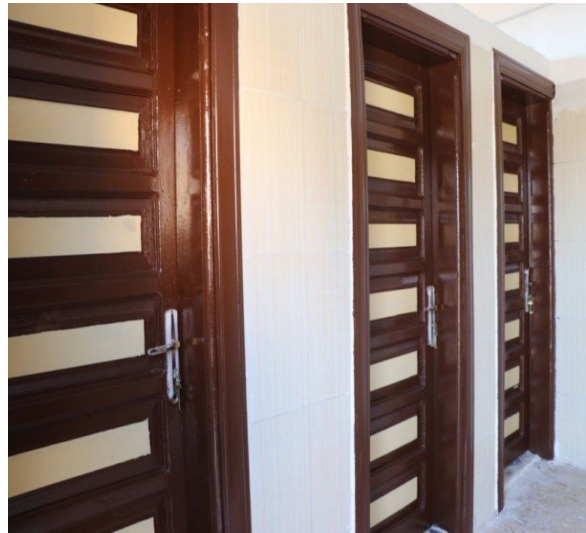
Aldahmash school following completed WASH rehab
