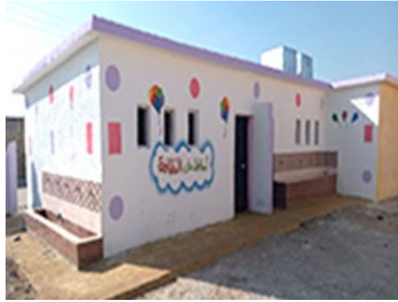
Alwahda school following completed WASH rehab
