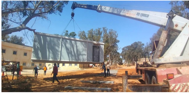
Mobile classroom installation in Abu Slim.
