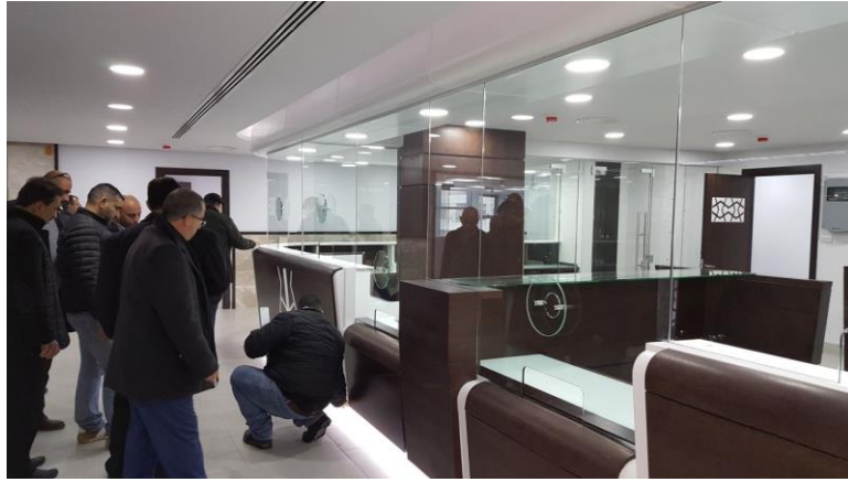
Final inspection of the newly renovated Nablus family court before handover.
